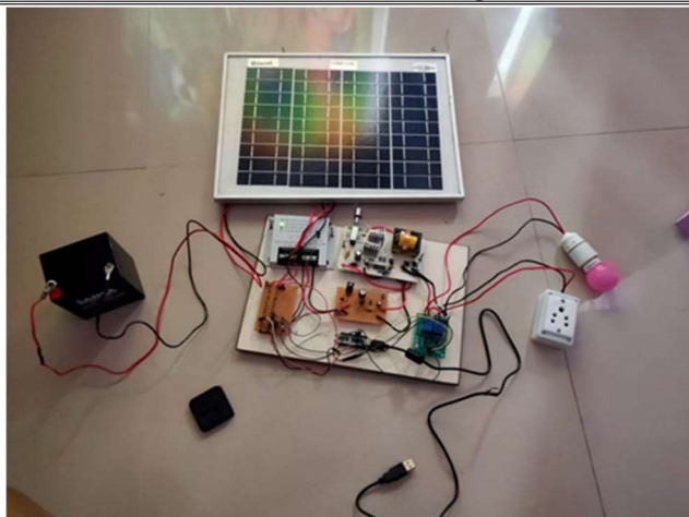
Fig. 13 Modelling of PV, Wind Battery system with Converter and Controller of Hybrid Energy Storage System.
